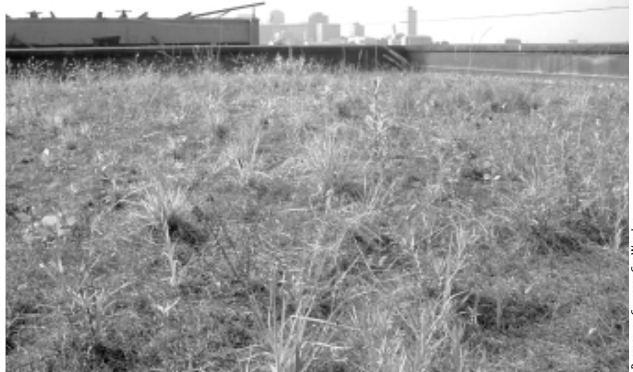
A view of the ecoroof in June 2003 looking towards downtown Nashville.
