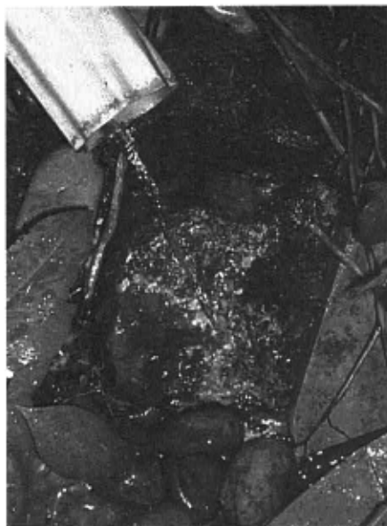
Deb Dale's north-side downspout
