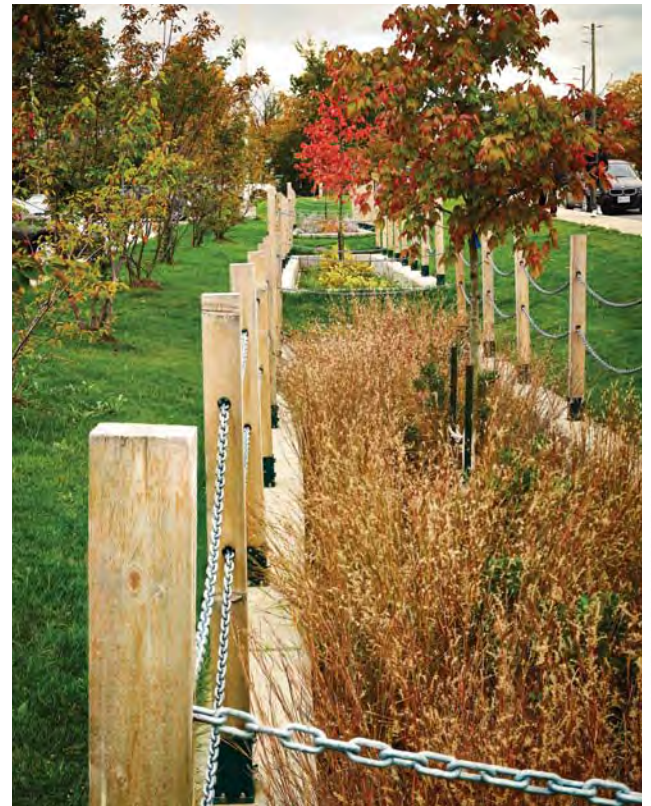
Elm Drive in Mississauga has been retrofitted according to LID practices. Rainwater is directed through permeable pavers into bioretention cells (rain gardens). In these cells, water is cooled and filtered before it infiltrates into the ground.
