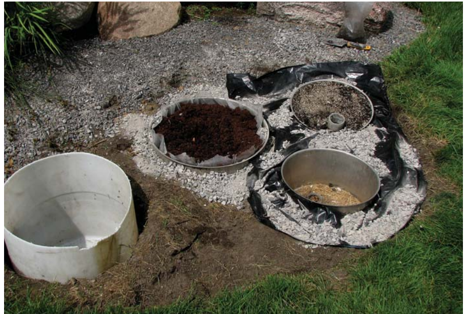
Installing containers on a slight slope in a low area. Gravel is laid on heavy plastic around containers.
