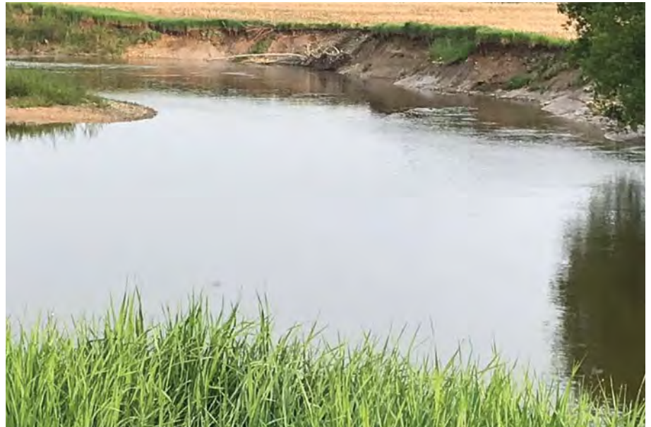
Riverbank erosion is exacerbated when land is cleared right to the edges.
