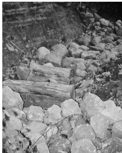
The hibernaculum under construction
