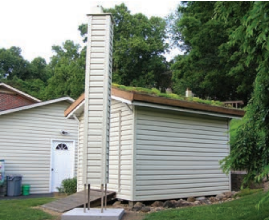
A completed chimney swift tower with the green roof of the shed just visible
