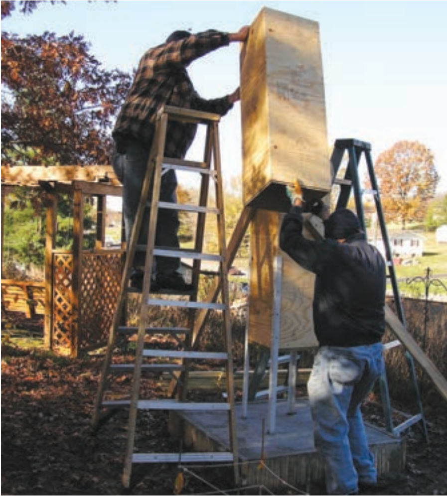
Building one chimney swift tower
